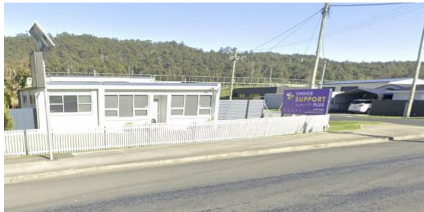
Figure 4 Existing street frontage, including sign
