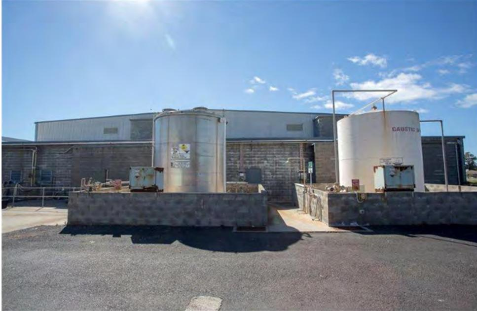
Photo 37 Hydrogen peroxide bulk tank (left) and sodium hydroxide bulk tank (right) (File Ref: AWM-28)
