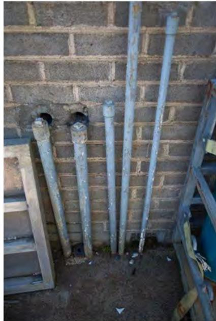
Photo 21 Blanked pipes on wall of welding bay/workshop. Pipe second from the right is the UST vent. (File Ref: AWM-66)
