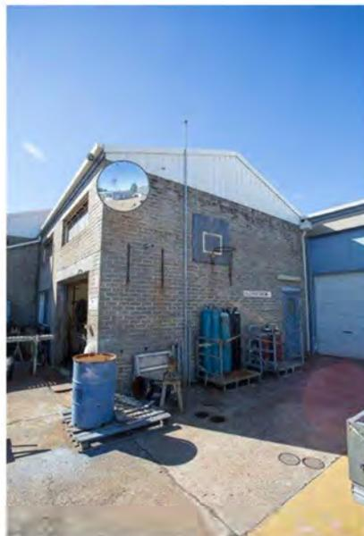
Photo 24 Welding bay/workshop, showing UST inspection ports and the UST vent on the wall (File Ref: AWM-4)
