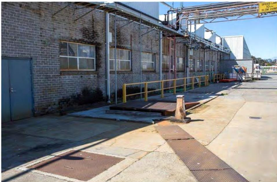
Photo 30 Staining on west wall of dye-house (File Ref: AWM-72)
