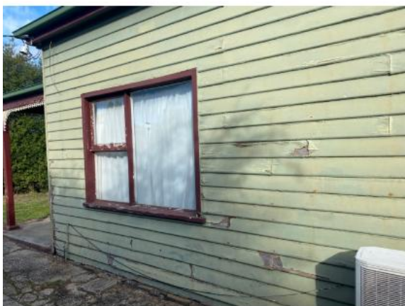
Figure 45: Some damage to boards. I would advocate window to be removed and wall weatherboard clad. Source: carste STUDIO
