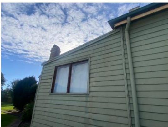
Figure 50: Aluminium window on south wall skillion section (Bedroom 3) showing the rotted architraves at the head. Source: carste STUDIO
