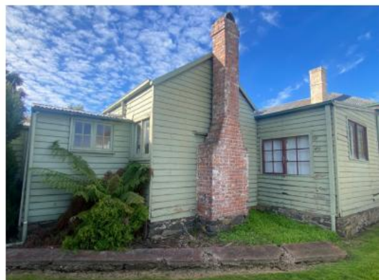
Figure 49: South western view showing (from right to left), Bedroom 3, Kitchen and chimney and Bathroom exterior. Bedroom 3 west wall boards are badly rotted. Note also the disconnected downpipe to the Bathroom. Source: carste STUDIO
