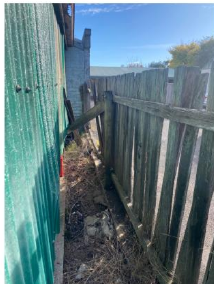
Figure 57: Carport north wall showing Alsynite cladding and north paling fence condition. Source: carste STUDIO
