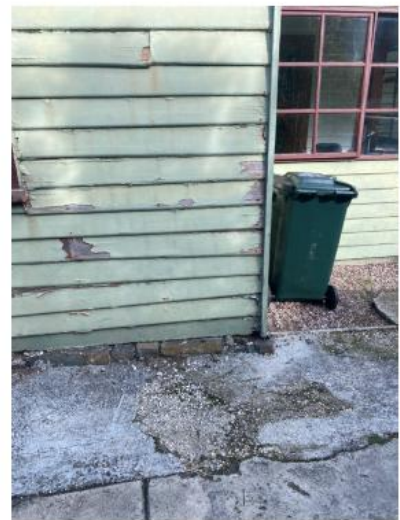
Figure 43: North wall west corner timber and paint decay Source: carste STUDIO
