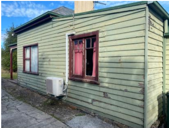
Figure 41: North wall has sustained the greatest deterioration Source: carste STUDIO
