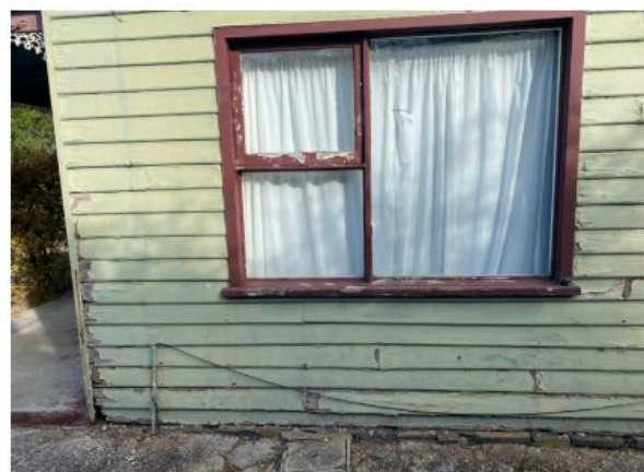
Figure 44: Some damage to boards. I would advocate window to be removed and wall weatherboard reclad. Source: carste STUDIO
