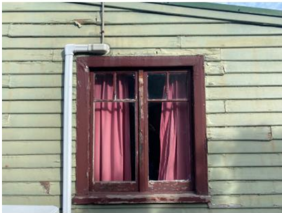
Figure 42: Northern Living Area window. Rot in window head and jamb boards and possibly lintel. Source: carste STUDIO
