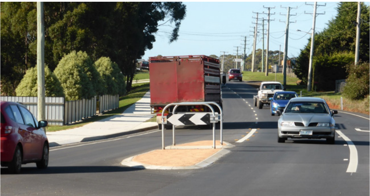
Figure 4: Completed project at Stony Rose Road, involving construction of pedestrian refuge, ramps and new path on northern (left) side
