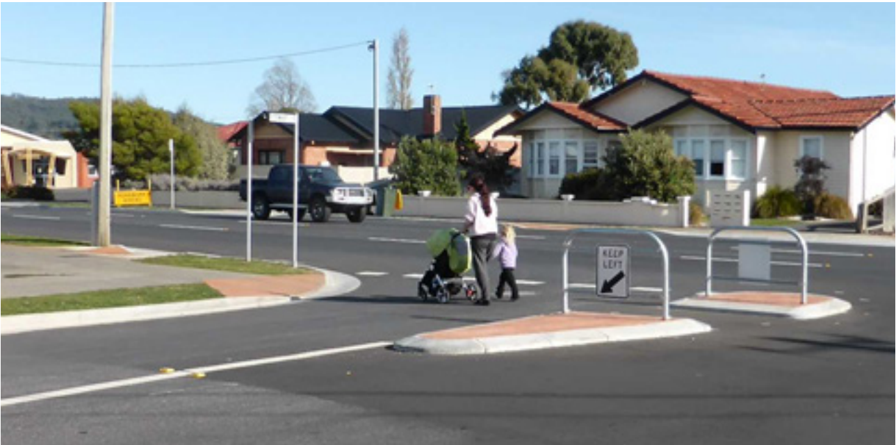
Figure 3: Completed project at William Street and Stewart Street, including construction of pedestrian refuge and ramps
