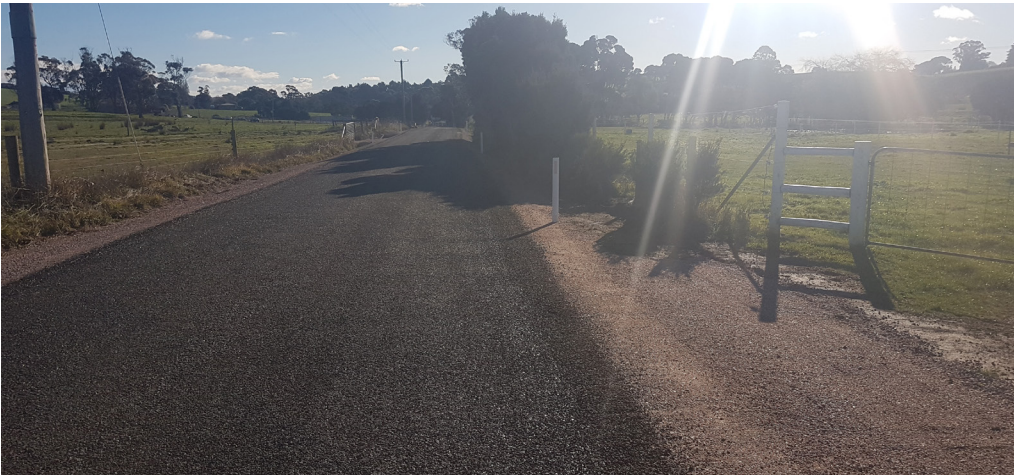
Stage 1 of the Winspears Road renewal was completed in March
