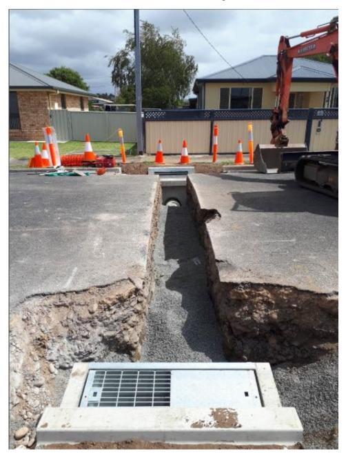
1.8. Work on the William stormwater catchment upgrade – stage 8 is almost complete. This project will alleviate local flooding issues. Construction was planned around major events at the Bluff over summer. Re-establishment of the grass on the Eugene Street field is now required before it can be used for winter sports.
