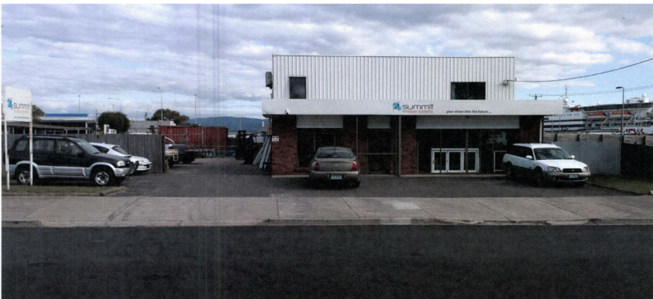
Figure 2 – Existing street view of 6-8 Thomas Street, East Devonport (Source: DCC – PA2016.0171).
