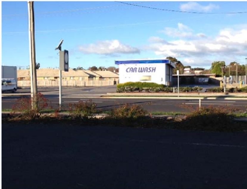
Figure 5 – Image of 114-116 William Street, Devonport
