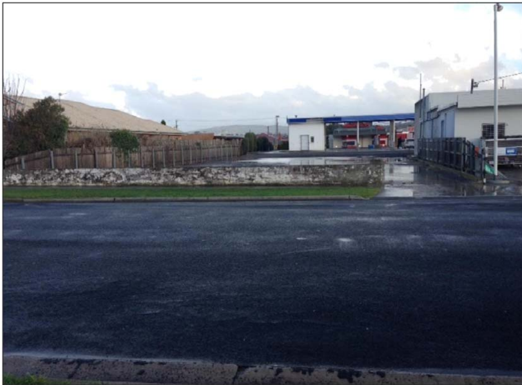
Figure 1 – Photo of 83 Stewart Street, Devonport
