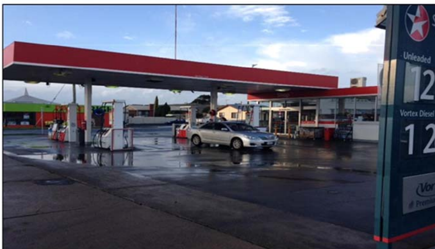
Figure 3 – Image of 118 William Street, Devonport
