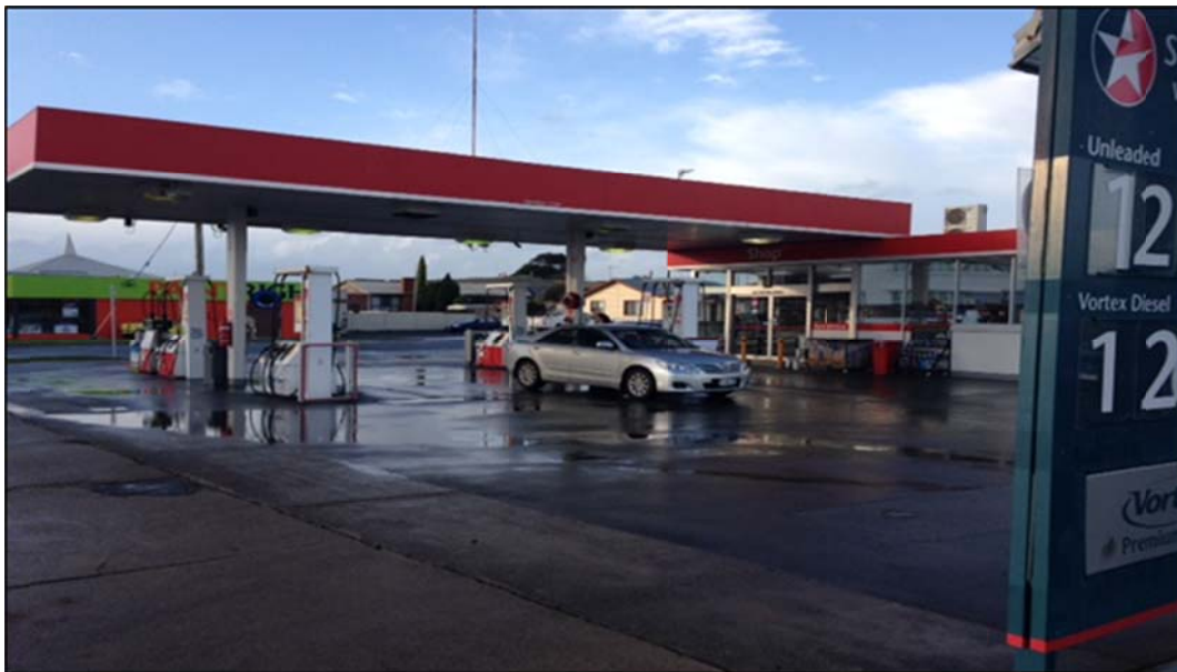
Figure 3 – Image of 118 William Street, Devonport
