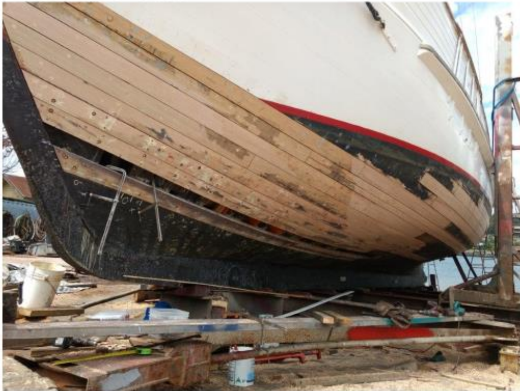
Extent of repairs – left side
