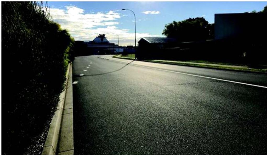
Figure 4 Wright Street towards Norton Way
