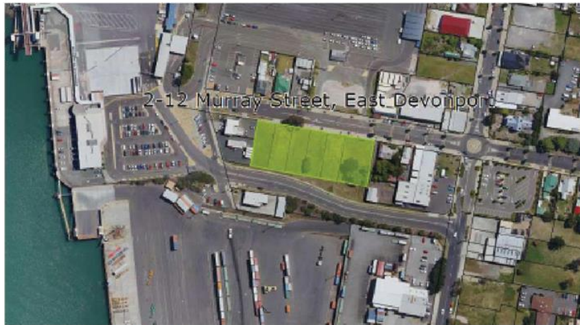
Image 1 - Aerial view of the site.
