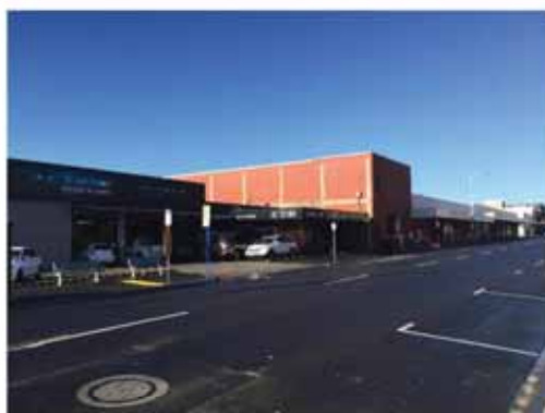
Figure 5: Existing Site from Rooke Street
