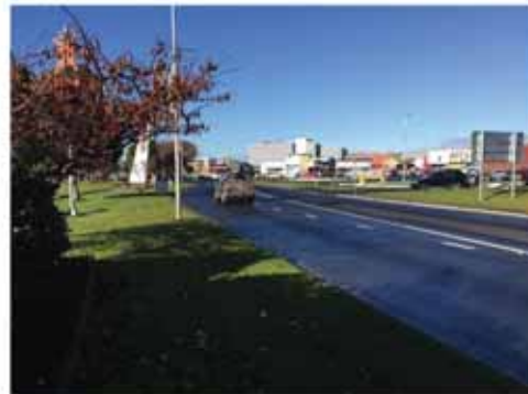
Figure 8: Formby Road (facing south)
