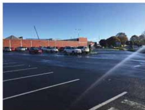
Figure 6: Existing Site from Formby Road
