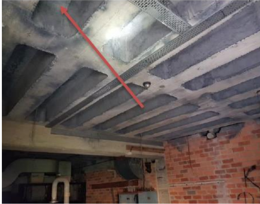
Photo 1 – ground floor void formers
