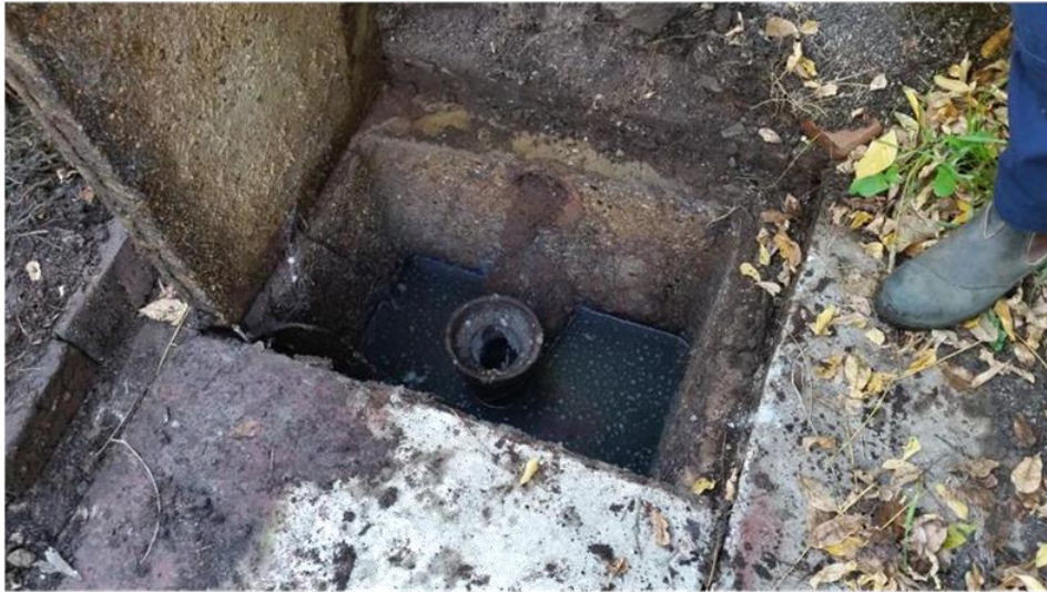
Photo 3. Septic tank outlet near carport
