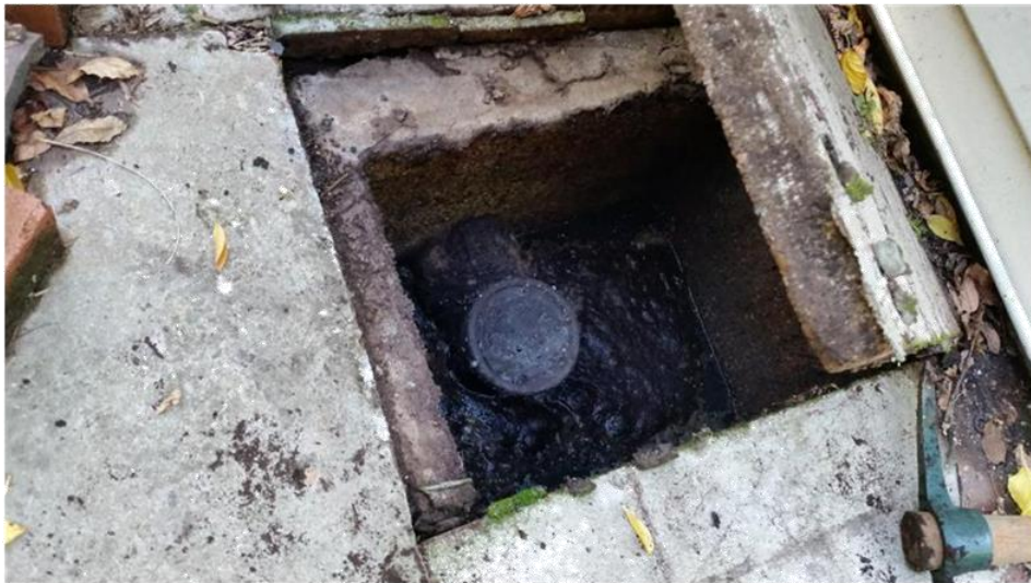
Photo 4. Septic tank inlet adjacent to house
