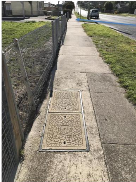
Figure 17 – Telecommunication services in the footpath along Tarleton Street
