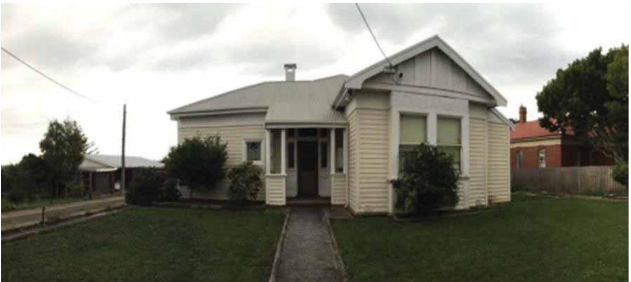
Figure 3 - Photo of existing building taken from Stewart Street (courtesy of Heritage Impact Statement by Tasmanian Consulting Service Pty Ltd 30/9/2016)
