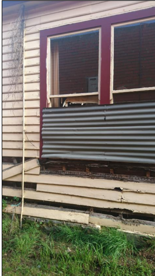
Figure 28 – 13 Victoria Parade – to be demolished
