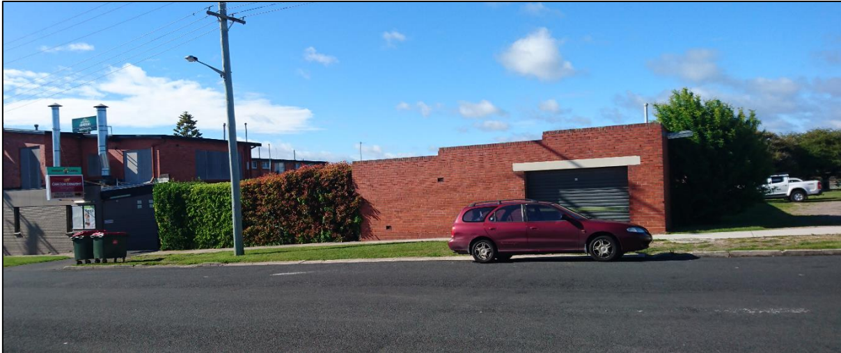
Figure 30 – existing motel accommodation (viewed from Lower Madden Street) – to be demolished
