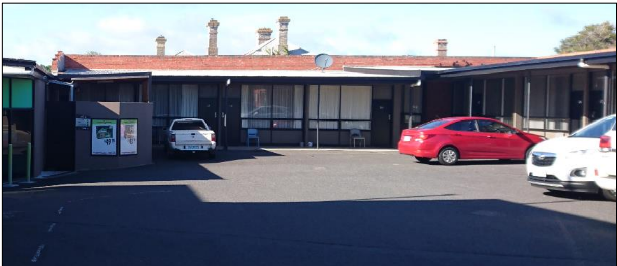
Figure 29 – existing motel accommodation – to be demolished
