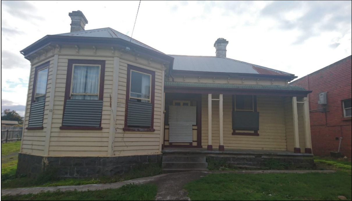
Figure 26 – 13 Victoria Parade – to be demolished
