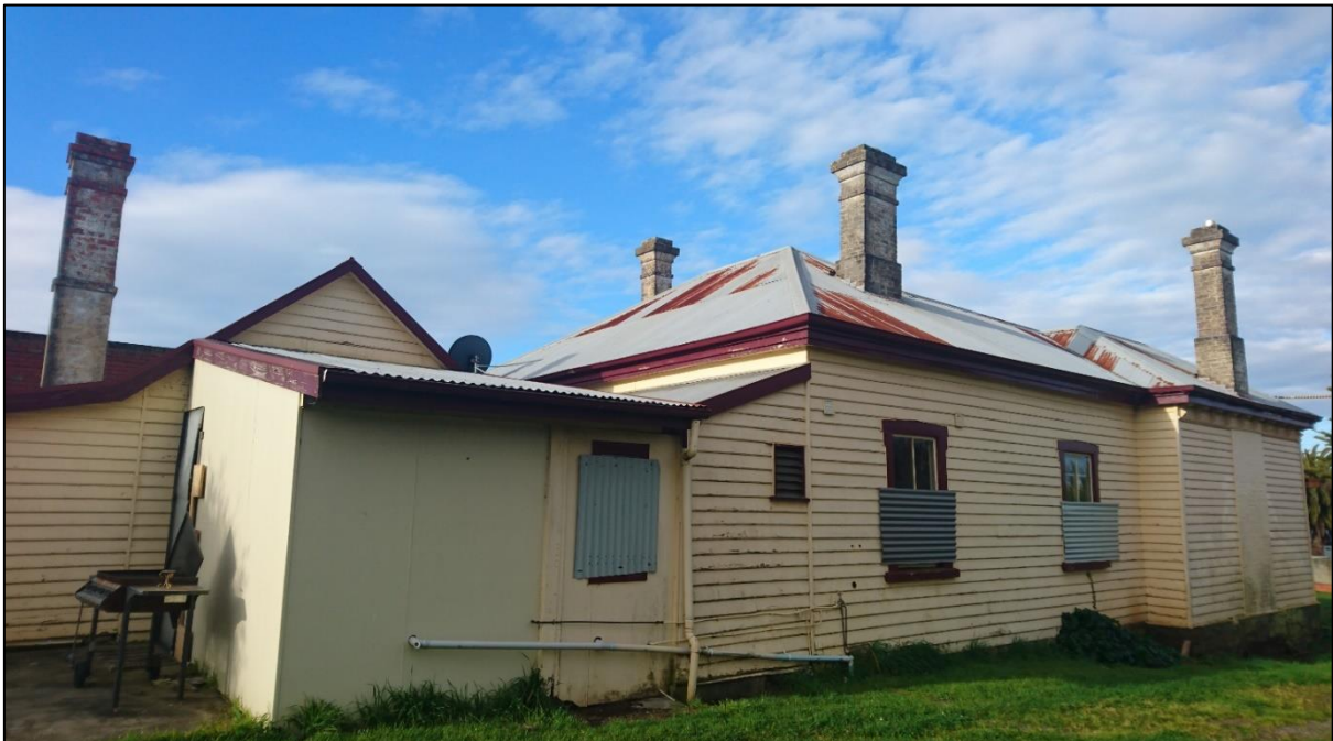
Figure 27 – 13 Victoria Parade – to be demolished
