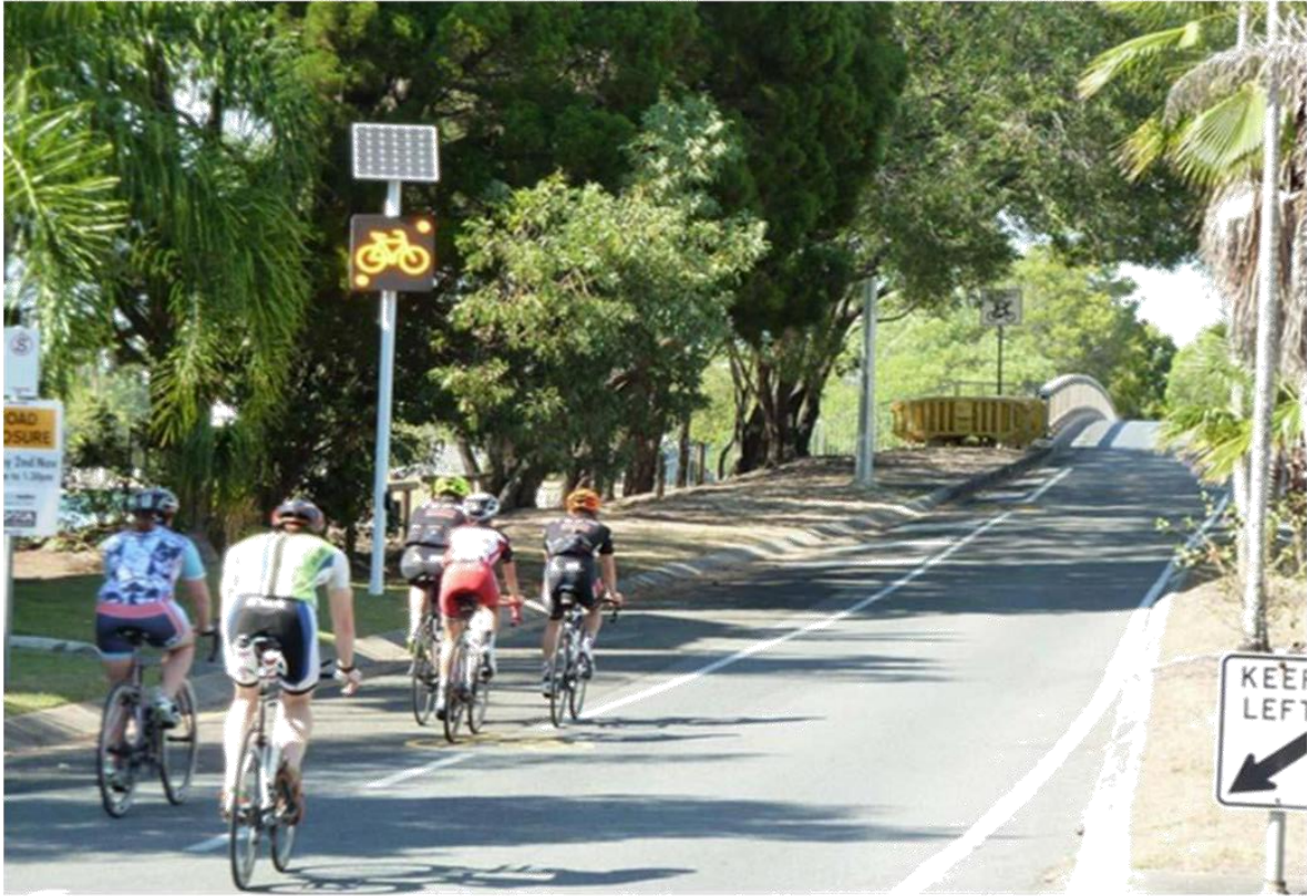
Munna Point Bridge, Noosa Heads, QLD
