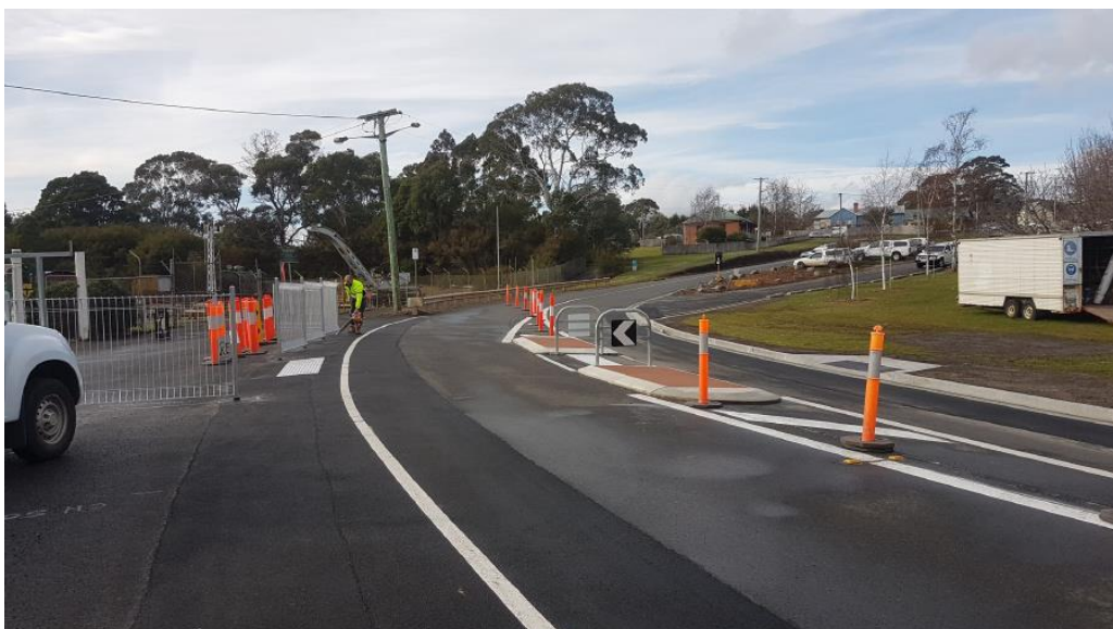
Forth Road project nearing completion (June 2018)
