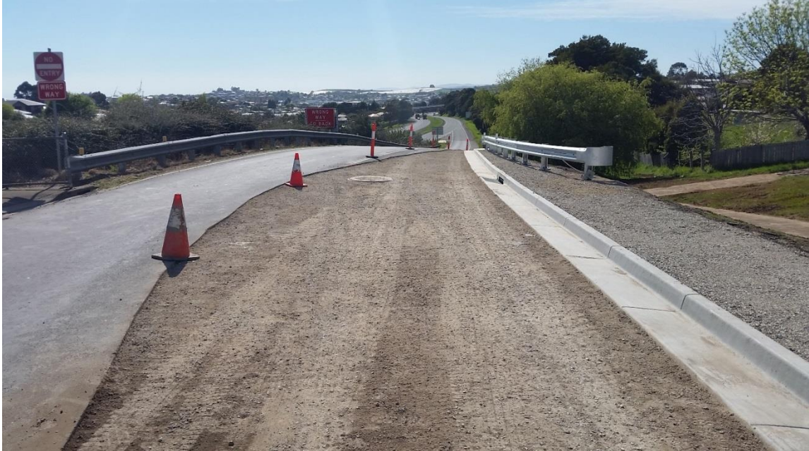
Middle Road west bound off ramp widening under construction (October 2017)
