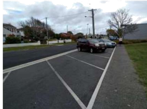
Figure 22: Parking Location B
