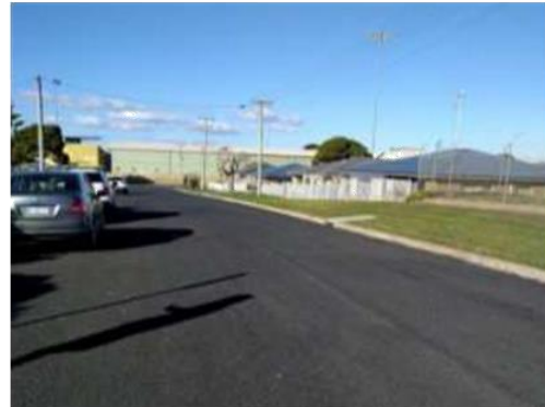
Figure 17: North Street near Meercroft Care (facing east)
