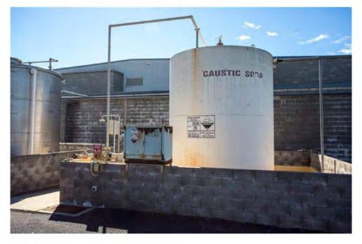
Photo 38 Sodium hydroxide bulk storage (File Ref: AWM-29)
