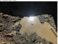
The water at the bottom of the UST pit had an oily sheen.
