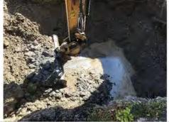
Oil soaked clay was present under the fill. The clay had a clear petroleum odour and distinctive black appearance. Water started forming at the bottom of the pit at 1.7 m.
