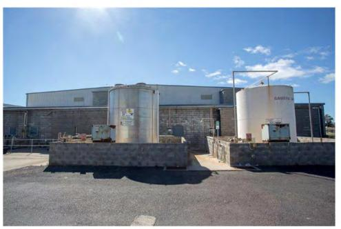
Photo 37 Hydrogen peroxide bulk tank (left) and sodium hydroxide bulk tank (right) (File Ref: AWM-28)
