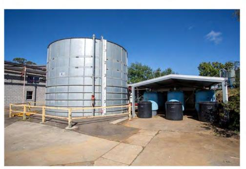
Photo 29 Fire tank (left) and covered storage (right) (File Ref: AWM-21)
