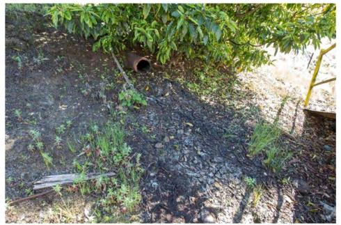
Photo 19 AST bund overflow pipe with staining on the ground (File Ref: AWM-70)
