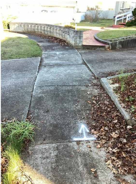
Pelion Place Footpath Replacement
