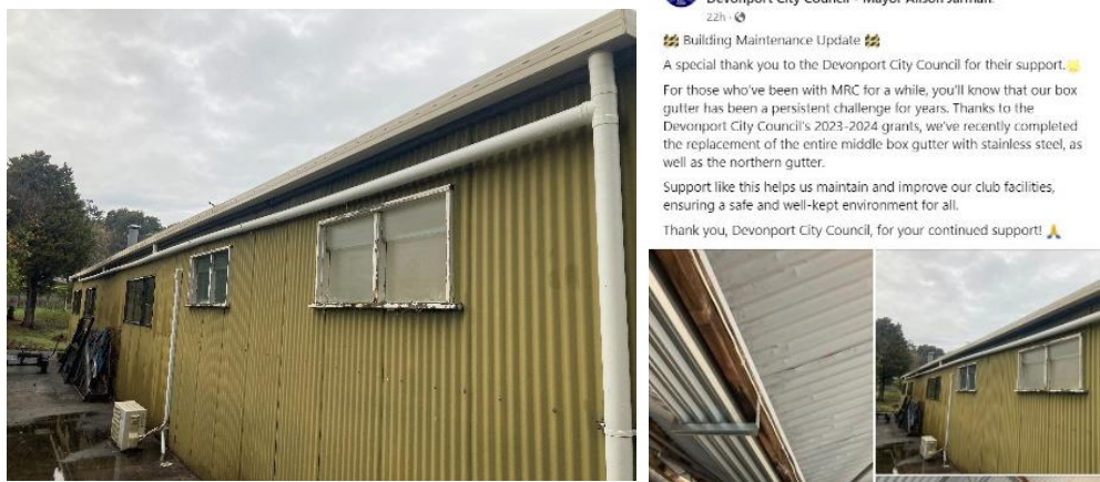
Roof repairs for the Mersey Rowing Club
