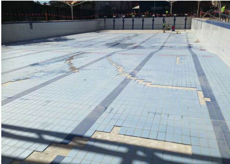
Example of pool floor tile delamination.
