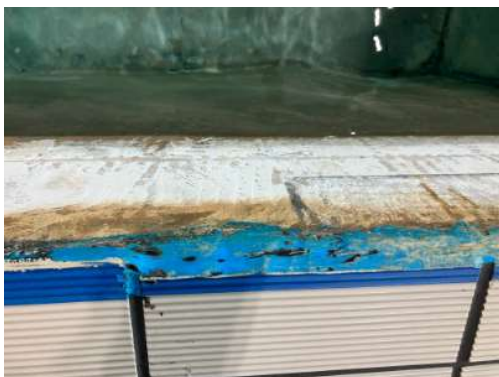
25m pool. Typical damaged edge tiles.
