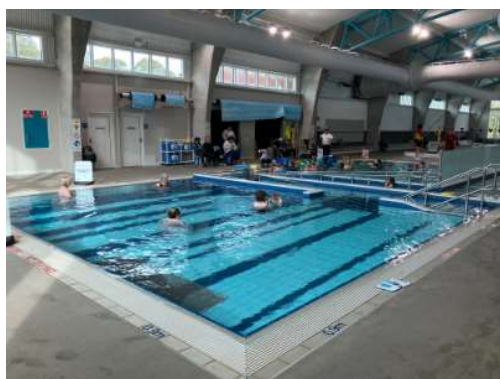
Leisure pool. Tiles missing on base at near wall.
