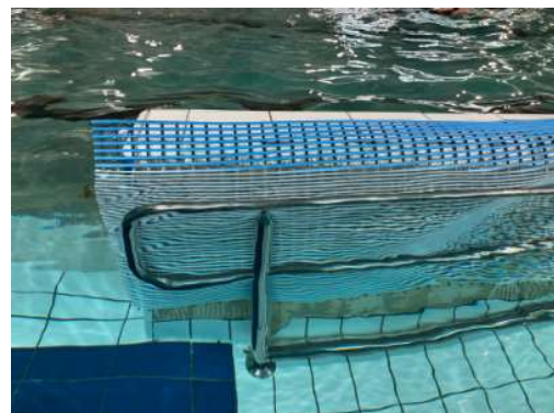
25m pool. Ramp section with failed wall tiles.
