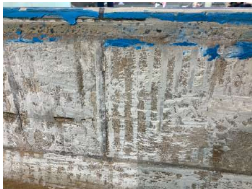
25m pool. Typical adhesive residue with notches.
