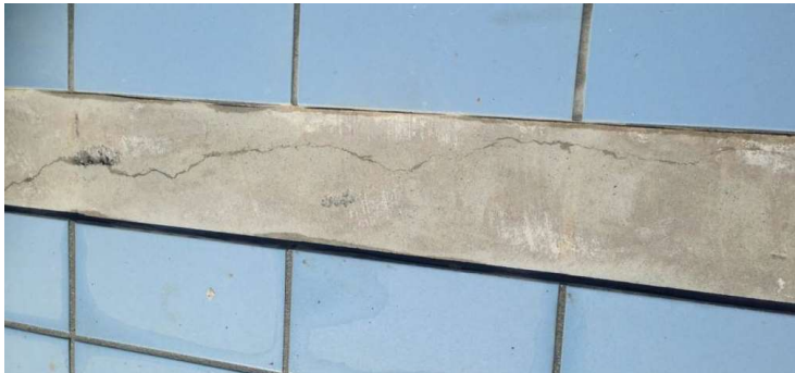
Example of concrete shrinkage crack not present before tiling, now present below row of failed pool tiles
