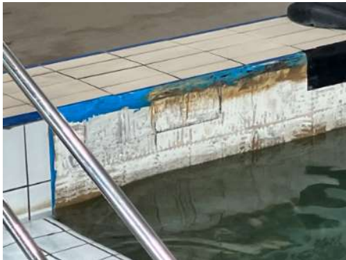
25m pool. Headwall tiles removed.
