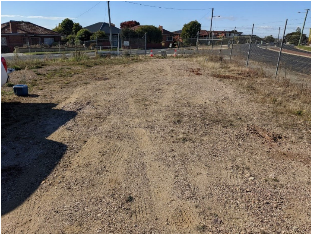
Photograph 9. Backfilled former tank pit
