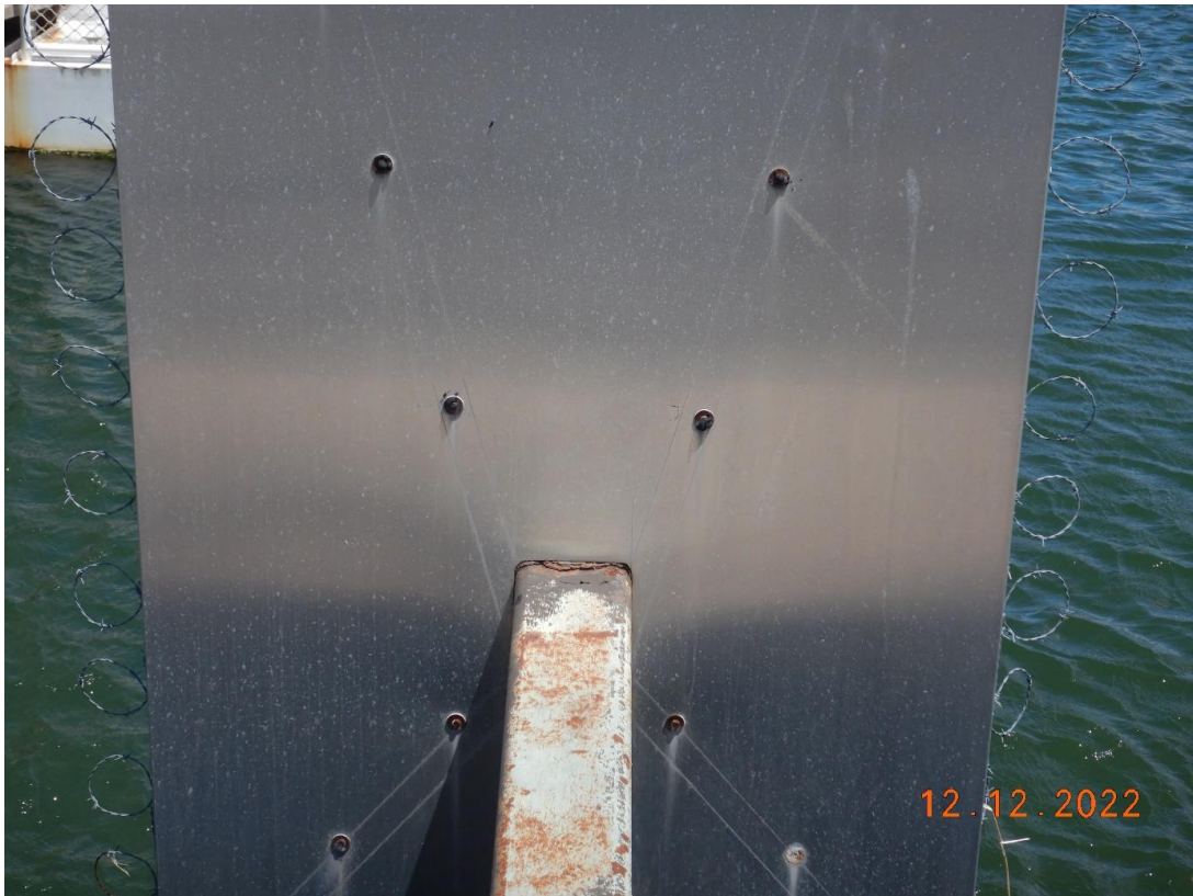
Isolated areas of Corrosion on Steel Truss Frame & Support Beams
