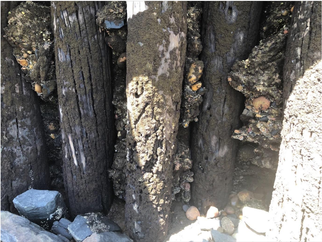
Failed Timber Pile at location of Gangway & Evidence of Teredo Worms Activity
