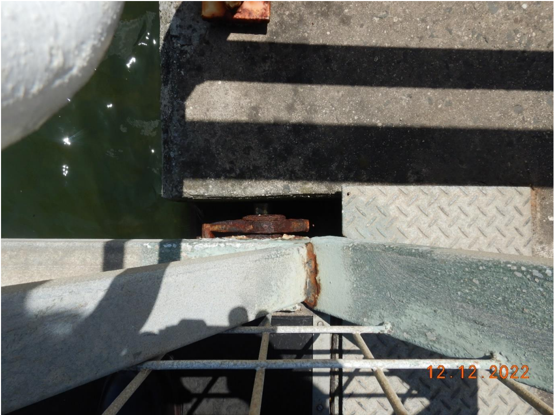
Severe Corrosion to Gangway Anchorage at Abutment
