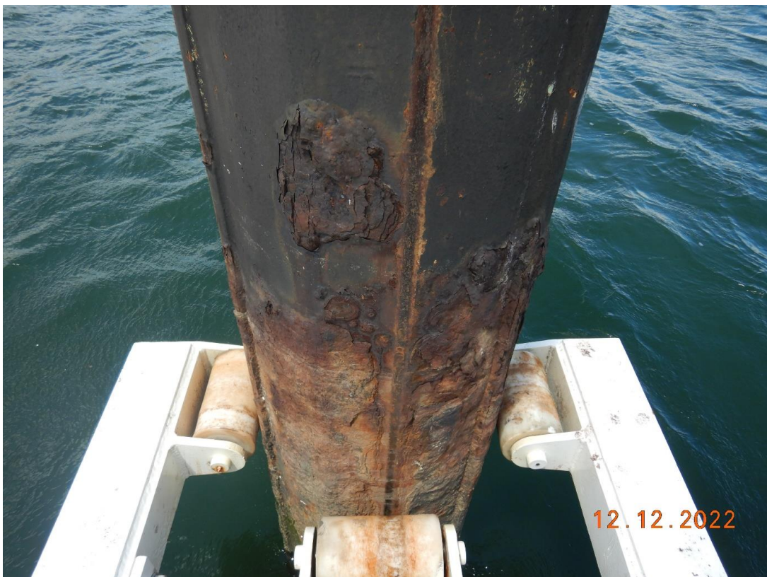
Severe Corrosion to Steel Piles now causing Section Loss
