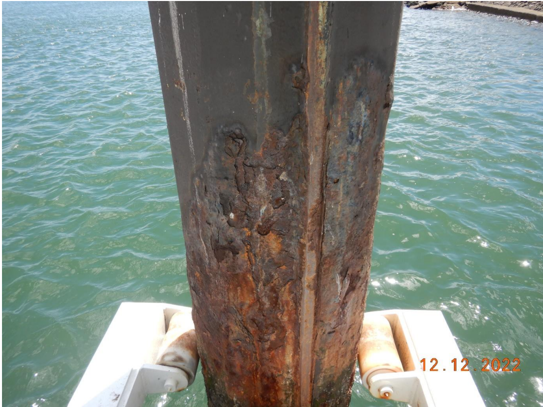
Severe Corrosion to Steel Piles now causing Section Loss
