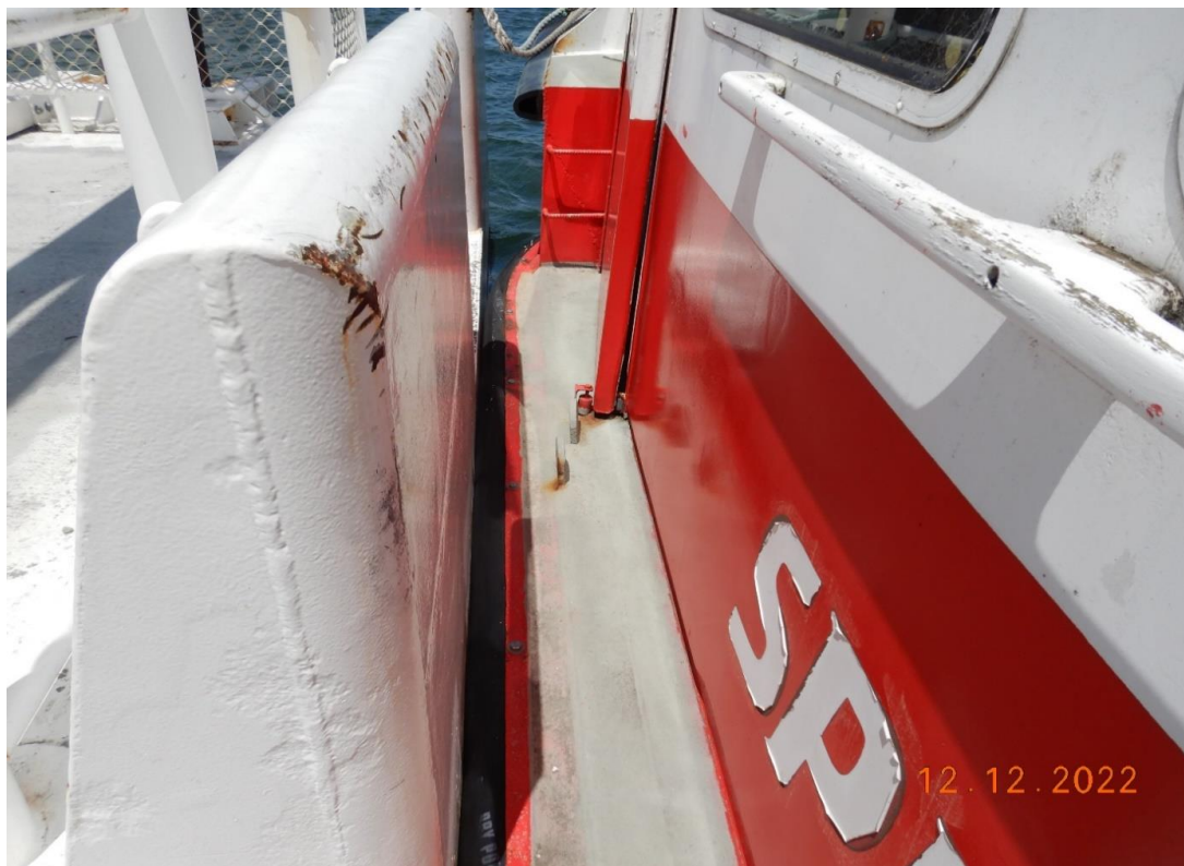
No Fender System installed along Pontoon Ferry Berthing Area
