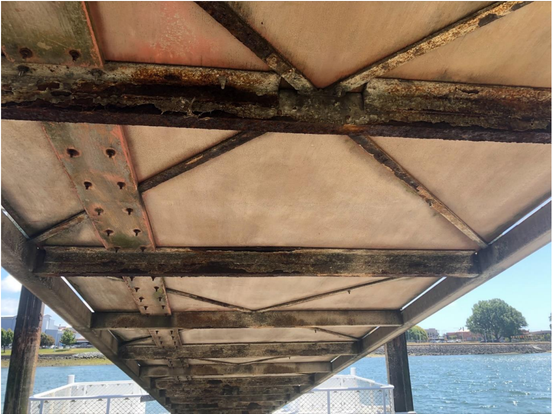
Severe Corrosion to Gangway Deck Support Beams
