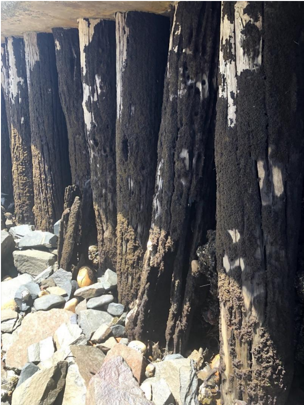
Failed Timber Pile at location of Gangway & Evidence of Teredo Worms Activity
