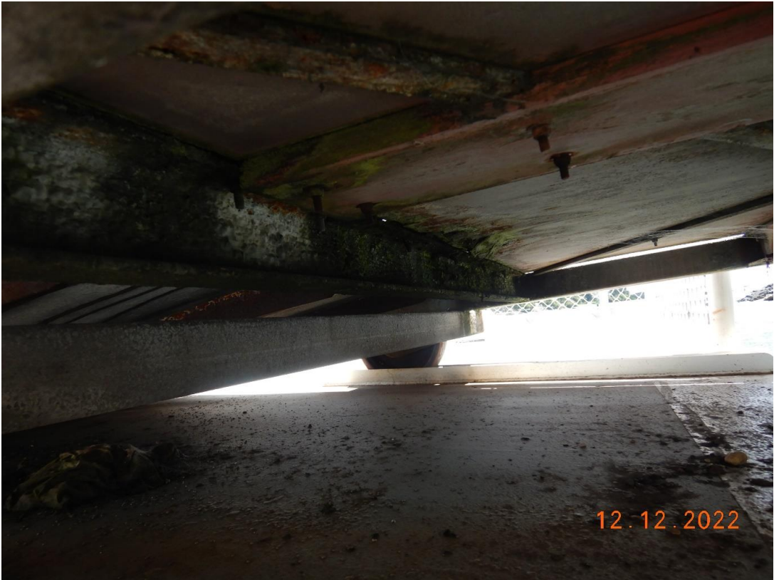
Severe Corrosion to Gangway Deck Support Beams
