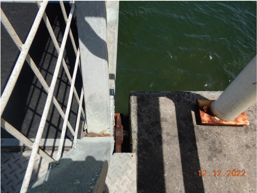
Severe Corrosion to Gangway Anchorage at Abutment
