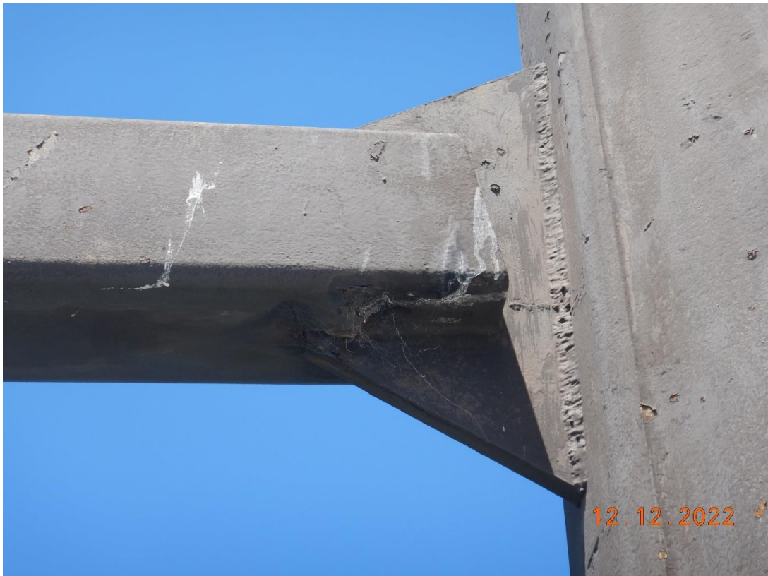
Isolated areas of Corrosion on Steel Truss Frame & Support Beams
