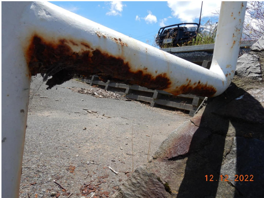
Failing bottom rail on Steel Pedestrian Barrier upstream due to Severe Corrosion
