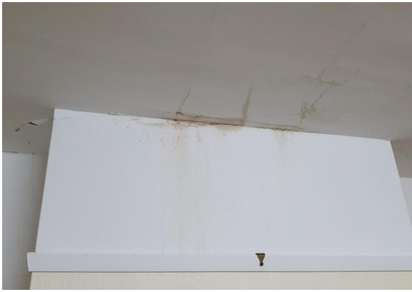
Inside the Annexe, showing cracking interior walls, and water damage around chimney.
