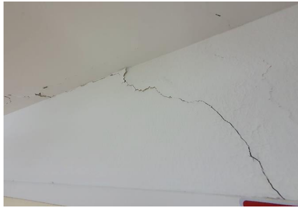
Inside the Annexe, showing cracking interior walls, and water damage around chimney.
