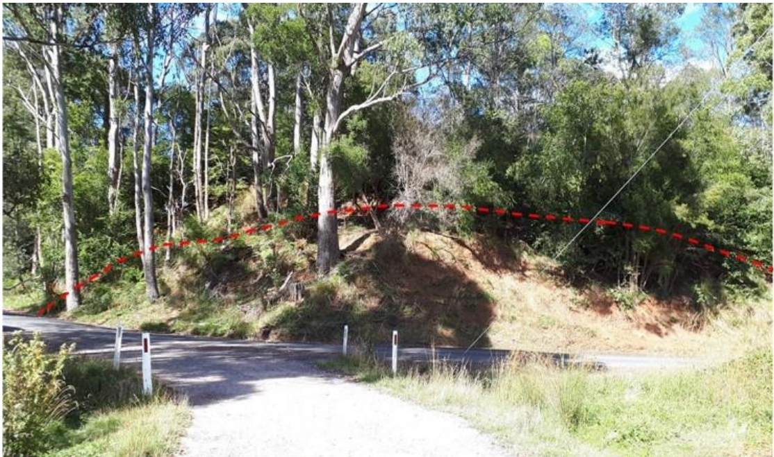
Lakeside Road – Works commenced on embankment to improve sightlines. Difficult site excavating in old quarry soils.
