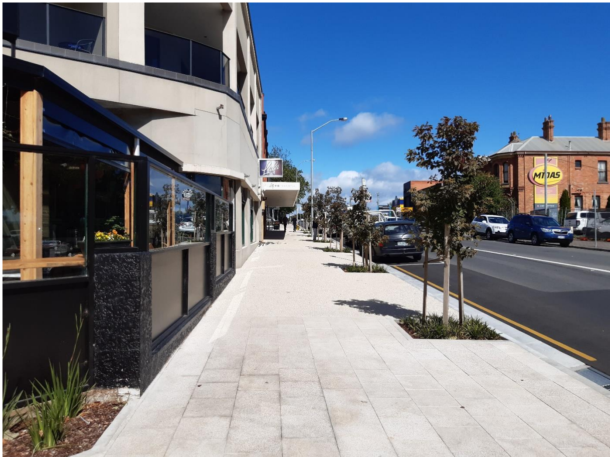
Oldaker Street – improved crossfall and width
