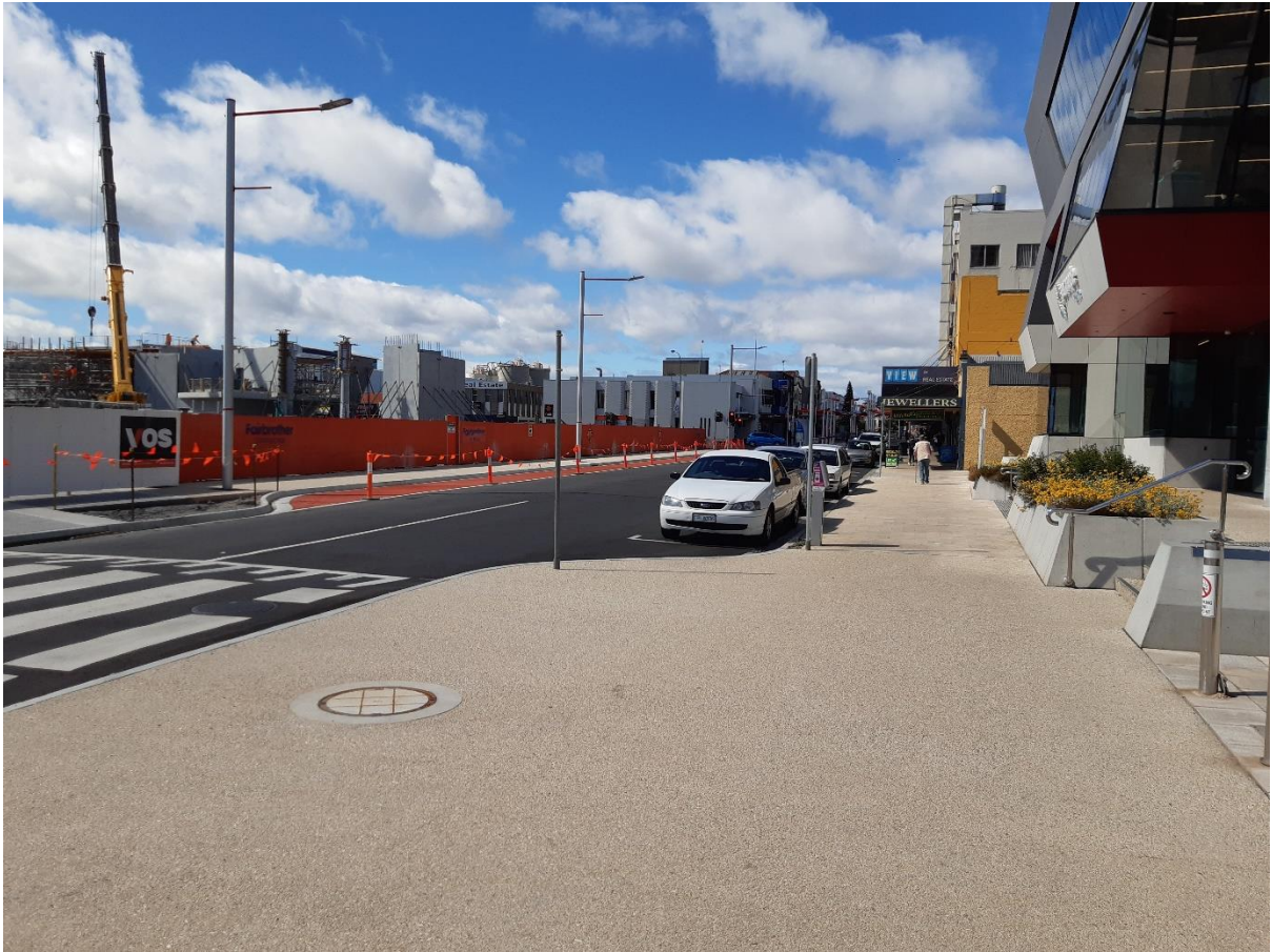
Rooke Street – Wider path with improved crossfall and priority 'wombat' crossing
