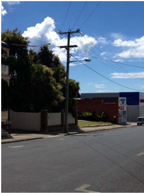
Figure 1 – Unmetered Lights on Aurora Energy Poles
