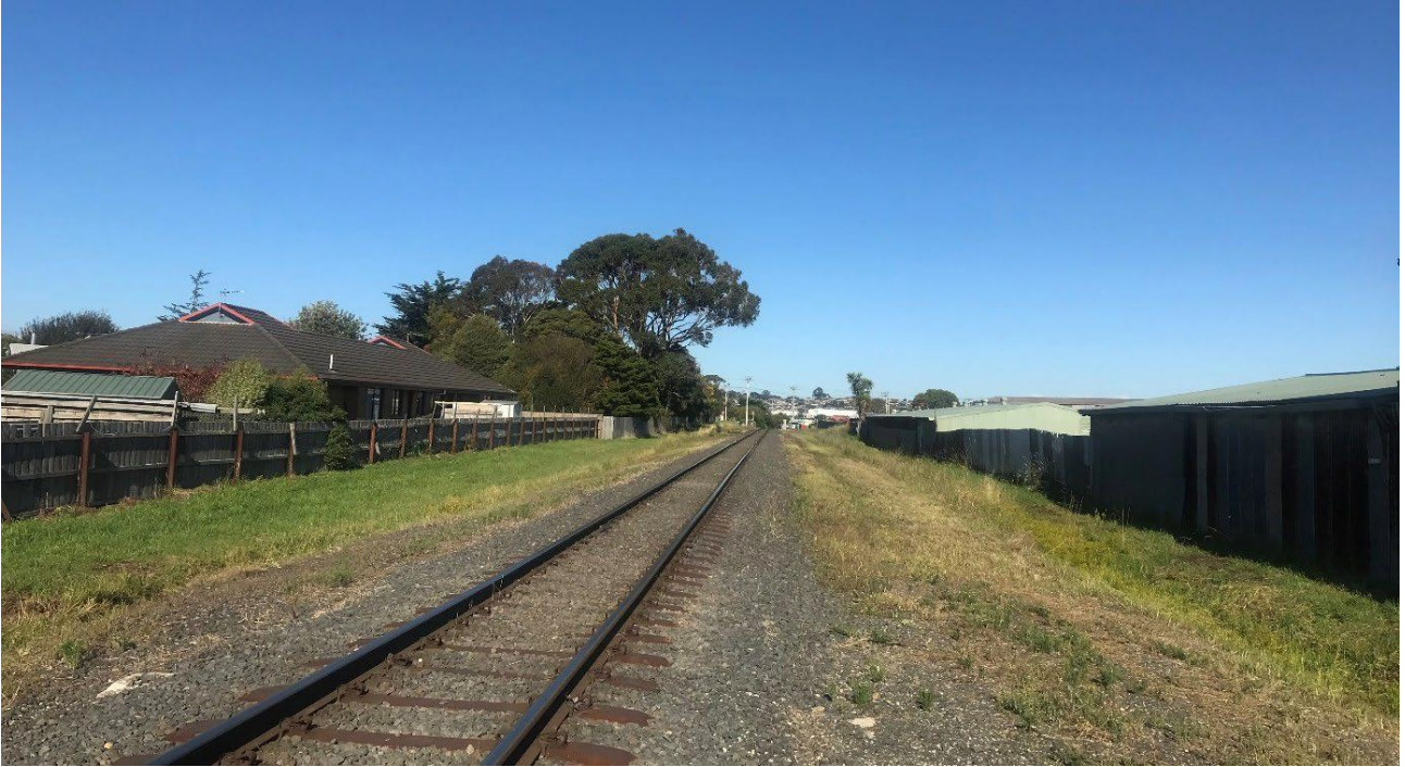
Figure 8: View of railway line looking south from Nicholls Street crossing (site on right hand side of image)
